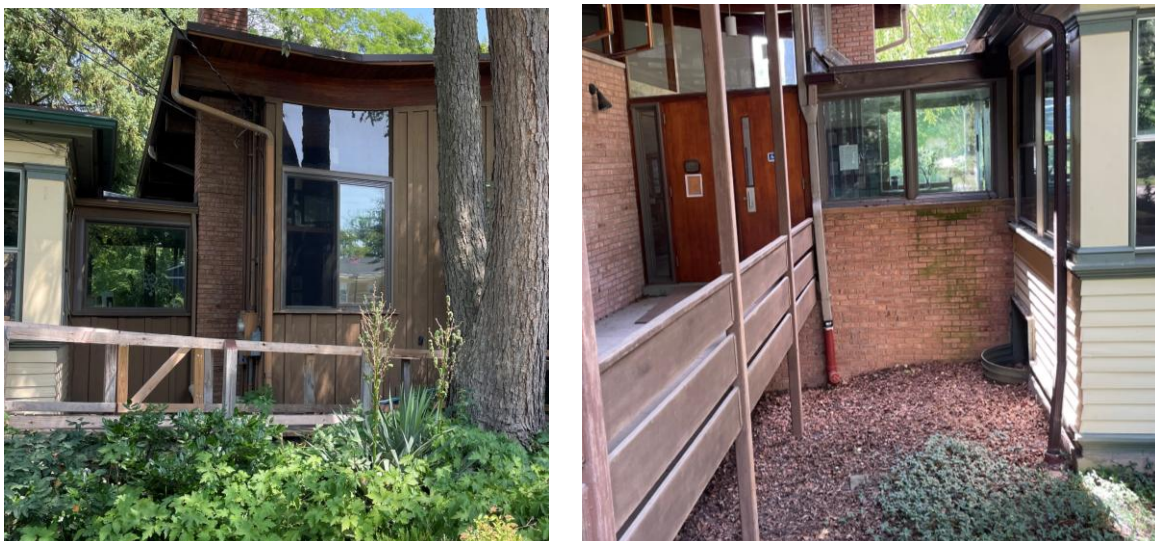
Figure 4: (Left) Space between buildings for outdoor unit. (Right) Space for second and future third outdoor units.
