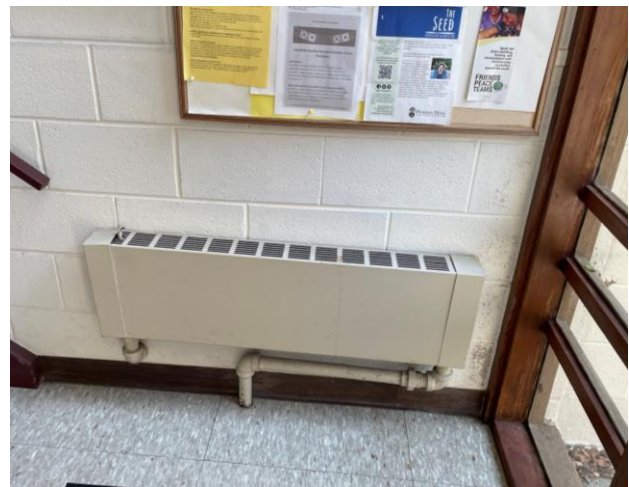
Figure 5: (Left) North wall of Meeting Hall. Replace finned tube radiator with cabinet unit heater (CUH). (Right) Entry finned tube radiator to be replaced with CUH.
